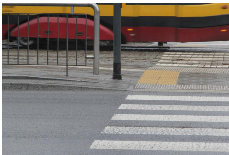
Pic. 1 Lowering the curb at the pedestrian crossing
